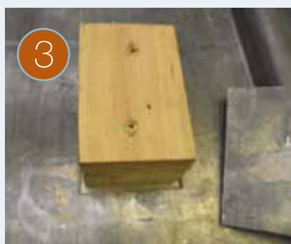
3 Support block secured to the roof structure, allowing 6mm gap for thermal movement when used on pitched roofs. Increasing the gap to 10mm would be advisable.
