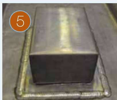
5 Lead capping piece with allowance for thermal movement where support rails/brackets can be fixed.
